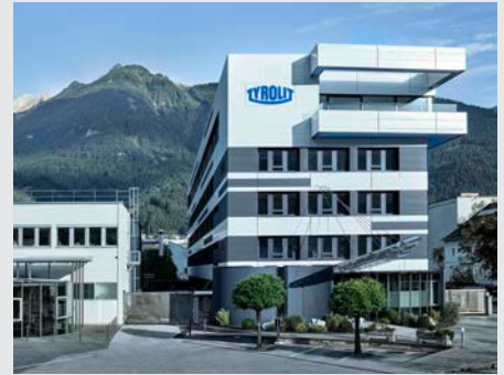
Tyrolit headquarters in Schwaz (Austria)
