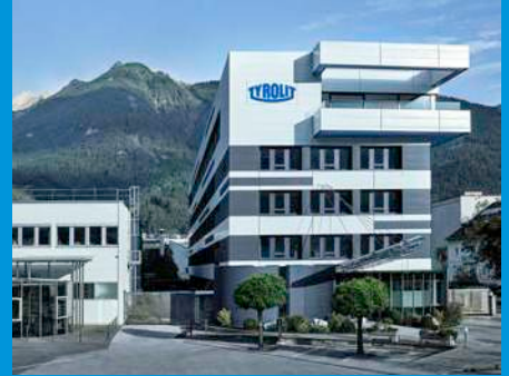
Tyrolit headquarters in Schwaz (Austria)
